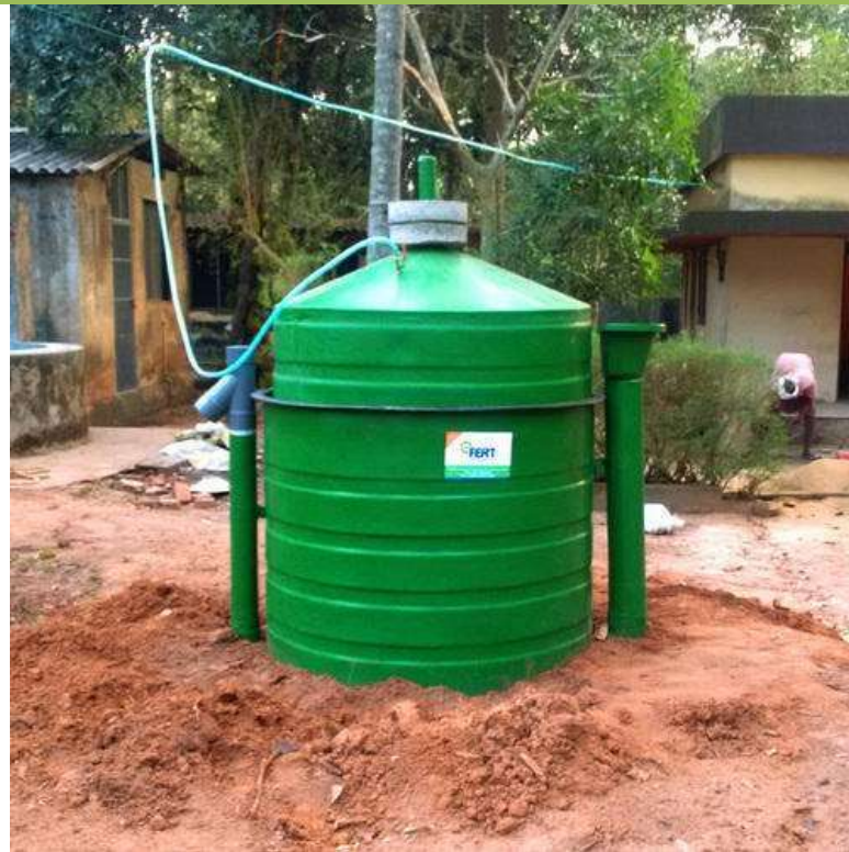
Bio-Gas Generation Plant - 10g/day- At canteen
